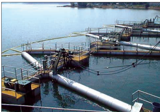
Figure 2. Improvements in Tennessee Valley Authority dam operations include (left) surface water pumps in the Douglas Reservoir (French Broad River, NC), designed to push oxygenated water from the surface to deepwater turbines, and (right) infuser weirs downstream of Chatuge Dam (Hiawassee River, NC), designed to provide both minimum flow and dissolved oxygen.
